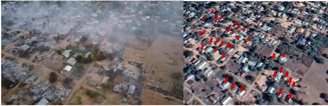
Figure 11: Images of fire and verification of structure damage in Tha Pyay Aye. Red icons indicate burnt buildings
