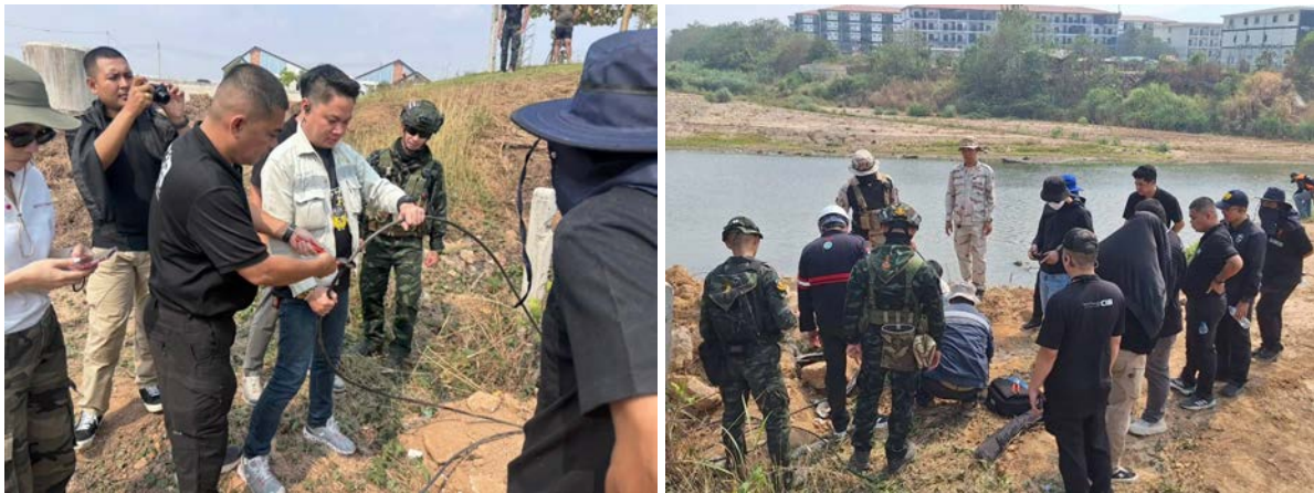
Figure 14: Thai authorities cutting internet cables and destroying suspected clandestine pipelines near Huanya Park, geolocated by Myanmar Witness to [16.650252, 98.523518] (Sources: [Left] KIC via Facebook, [Right] จังหวัดตาก 24 ชั่วโมง via Facebook).
