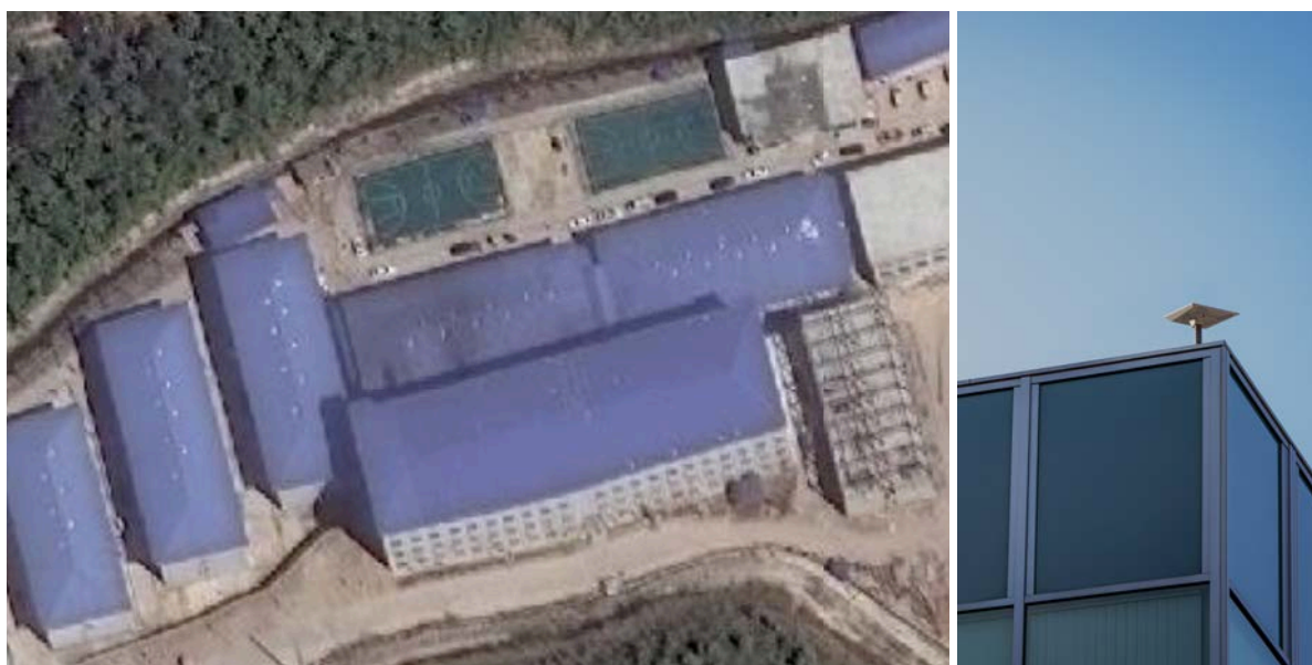
Figure 11: Qingsong Park [16.427589, 98.63444] appears to have Starlink devices attached to the roofing already, as observed in high-resolution imagery (Sources: © 2025 Vantor) [Right] Starlink ).
