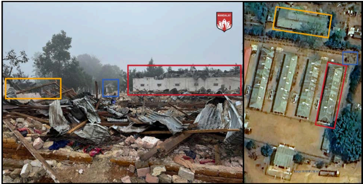
Figure 25: [Left] UGC shows damaged buildings after an alleged airstrike on Ho Hko Labour camp [22.392634, 96.523068]. (Sources: [Left] MDY-PDF , [Right] Google Earth imagery @2026 Airbus)
