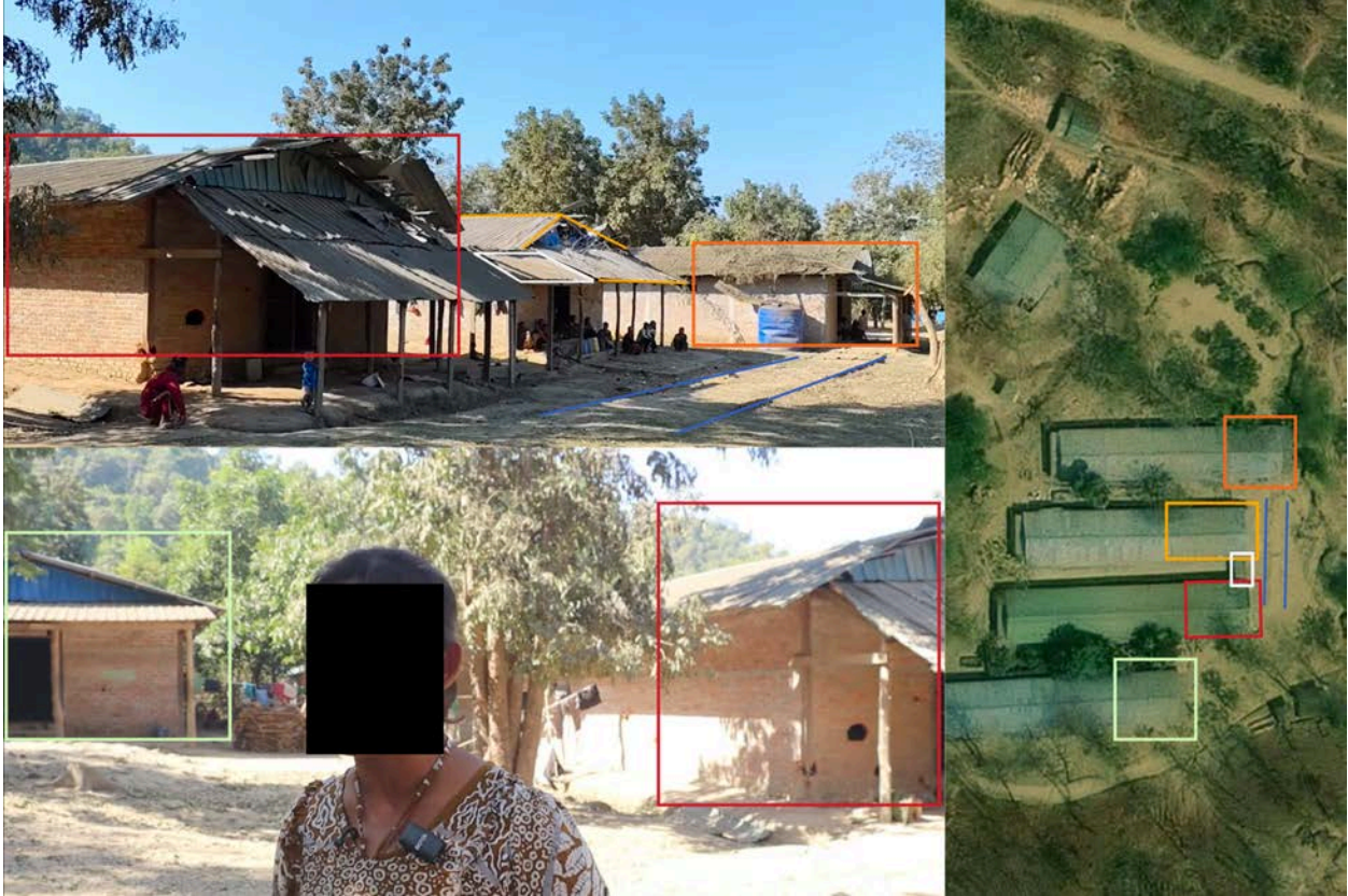
Figure 21: Geolocation of the damaged site at [20.648250, 92.911829] (Sources: Burma News International via Facebook & © Apple Maps, 2026, Maxar Technologies)
