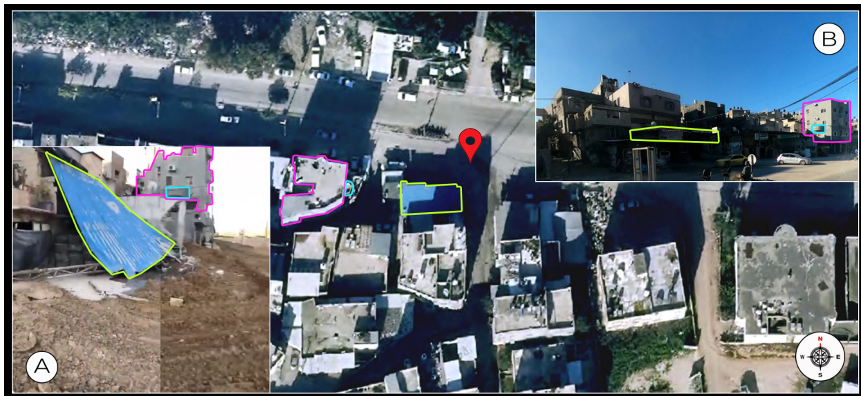
Figure 13: CIR geolocated road infrastructure damage in Nour Shams refugee camp, Tulkarm, at coordinates: 32.3192, 35.0631. Sources: Geomolg, A: IP2618 and B: Mapillary. 72
