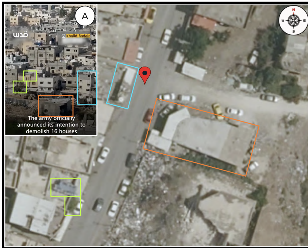
Figure 25: CIR geolocated road and residential building damage in a residential area of Tulkarm, at coordinates: 32.3136, 35.0371. Sources: GovMap, A: IP11485. 114
