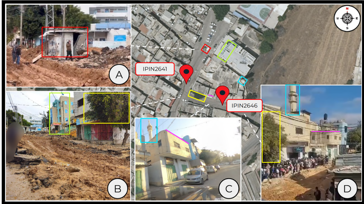
Figure 18: CIR geolocated damage and ISF presence on al-Fara'a Road, al-Fara'a refugee camp, at coordinates: 32.2918, 35.3451 (IPIN2641) and 32.2918, 35.3454 (IPIN2646). Sources: GovMap, A: IP10690 and B: IP10627, C: Mapillary, D: IP10719. 137
