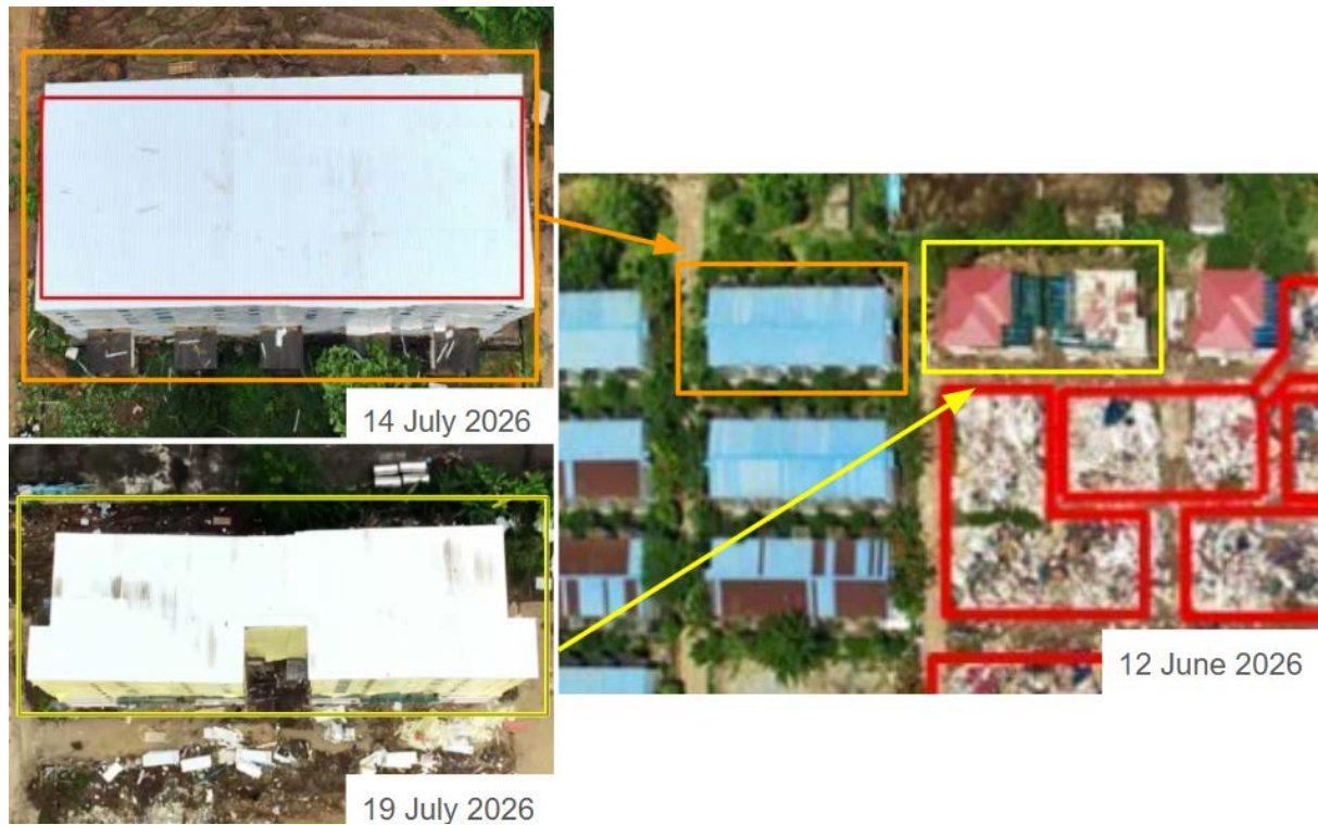
Figure 11: [Top Left] Image of the 14 July 2026 building showing no roof and a taller build [16.820846, 98.538977] (source: 妙瓦底论坛 | 妙瓦底新闻 | 亚太新闻 | 缅甸新闻 ); [Bottom Left] Image of the 19 July 2026 building showing a taller build [16.821149, 98.538964] (source: MRTV ); [Right] Zoomed-in imagery of the two buildings showing original roofs from 12 June 2026 (source: 妙瓦底论坛 | 妙瓦底新闻 | 亚太新闻 | 缅甸新闻 ).
